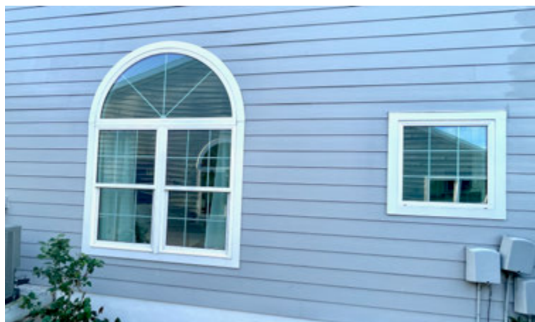
Grand Cayman Palladian window and new window with grids (former Garden window).
